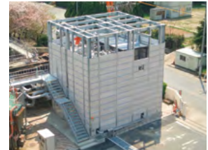
Sludge treatment facilities
