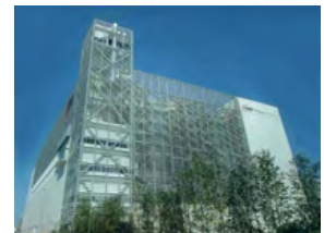
Waste treatment facilities
