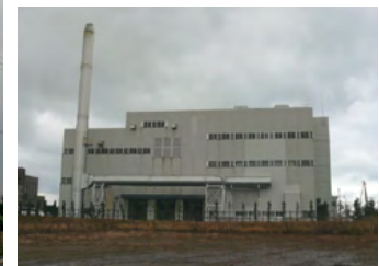
Building on which a temporary steel stack was installed (after the disaster recovery)
