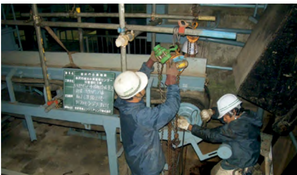
Recovery work (checking and installing the motor)
