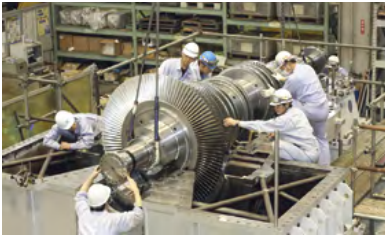
Steam turbine assembling work
