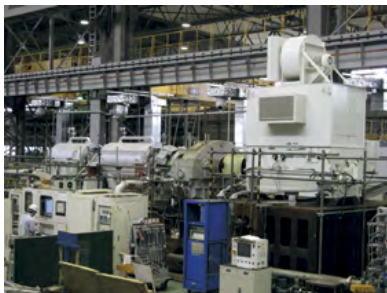
Electric motors and compressors at test facility
