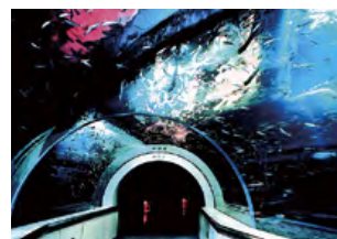
Water treatment facilities for aquariums
