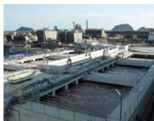
Plant wastewater treatment facilities
