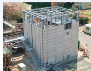
Sludge treatment facilities
