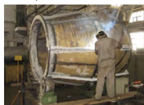
Welding of discharge bowl at EQC
