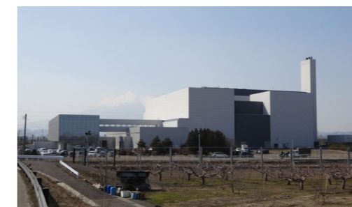
In the fiscal year ended March 31, 2016, we received an order for the long-term comprehensive management of Hiroasaki Area Environmental Maintenance Center, shown above.
