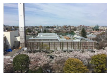
Waste incineration plant with electricity generation facilities (Musashino Clean Center)
