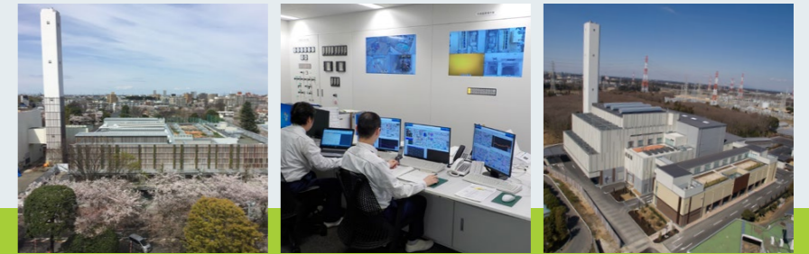
(From left) Musashino Clean Center completed in March 2017 Central control room of waste incineration plant Funabashi City north waste incineration plant completed in March 2017
