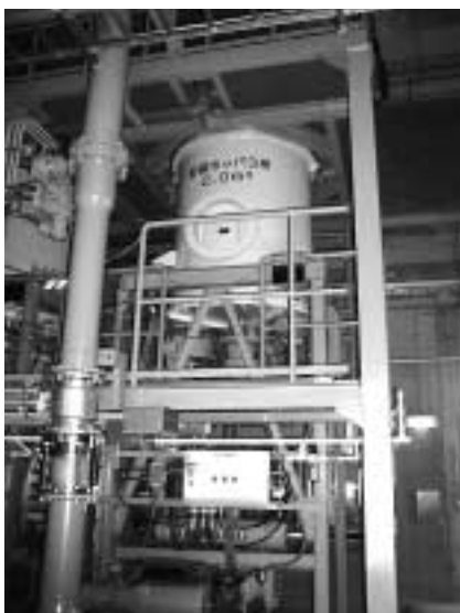
写真34 臭素系消毒設備 Photo 34 Disinfection system
