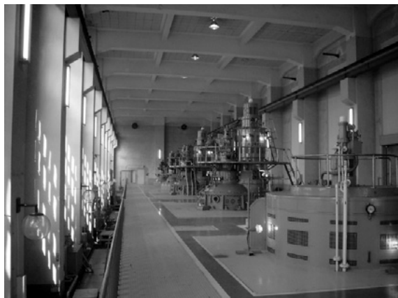
改修前ポンプ室内全景 Driver room before renovation
