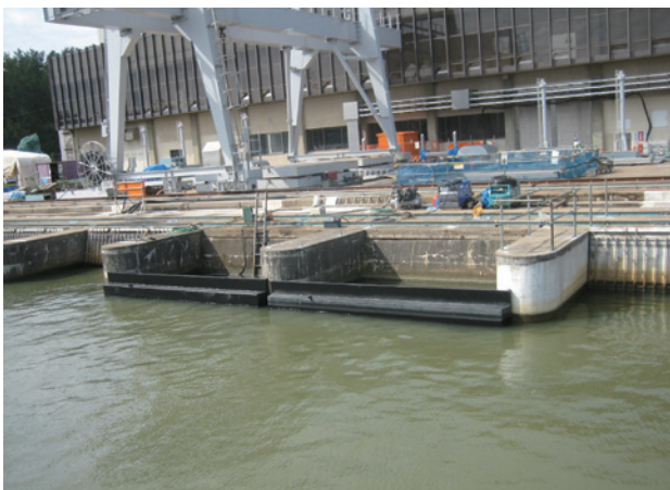
写真2 吸込水路の仮止水壁設置状況 Photo 2 Setting up stop-log at suction channel
