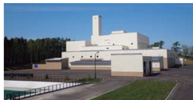
Garbage incineration facility constructed for Iwamizawa City, in Hokkaido (Iwamizawa Environment Green Plaza)
